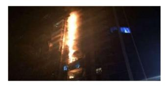
"Flames spread rapidly up the external wall cladding at the Lacrosse building in Melbourne in November 2014. More than four years on, the combustible panels were still in use".
