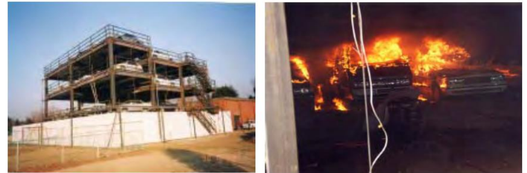
FIGURE 1. The external view of the experimental structure and the view of the spreading car fire during the experiment
