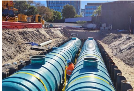
KSA Hangar Foam Containment Storage [image courtesy Atlan Stormwater (2026)]
