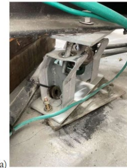
Rooftop diesel generator – vibration mounts without lateral restraint capacity.
