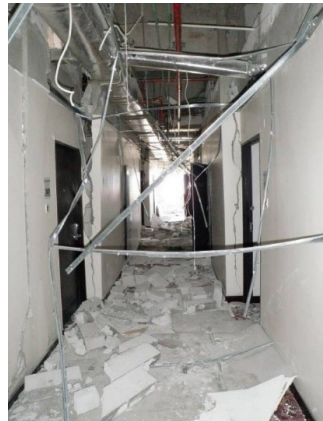
5. Ceilings crushed
