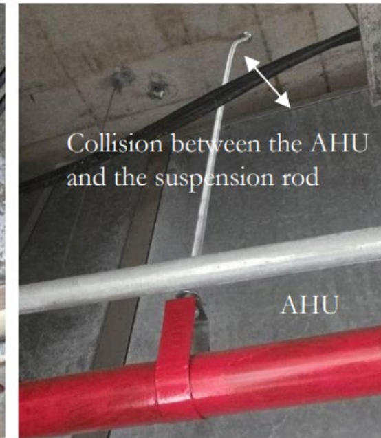
Figure 8. Suspension rod
