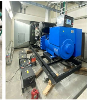
Rooftop diesel generator – vibration mounts without lateral restraint capacity.
