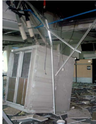
2. Support failure
