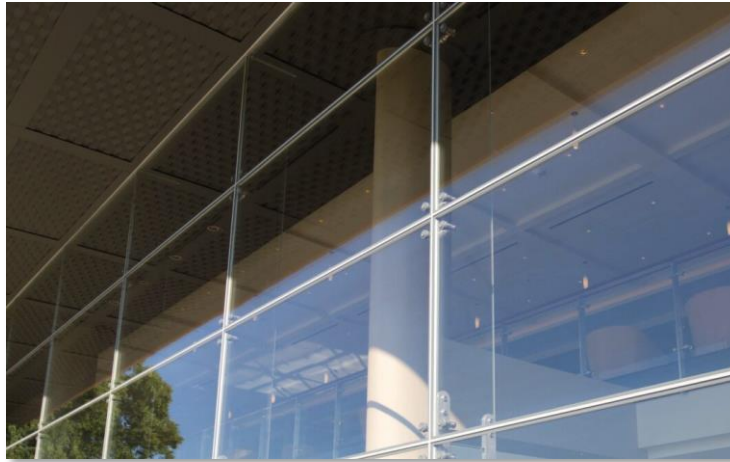
Pressure Wall / Structural Glazing
