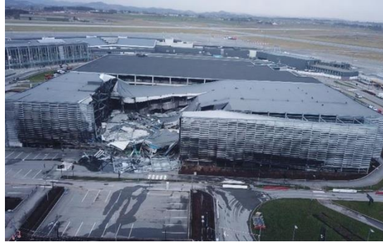
Stavanger Airport, Norway
